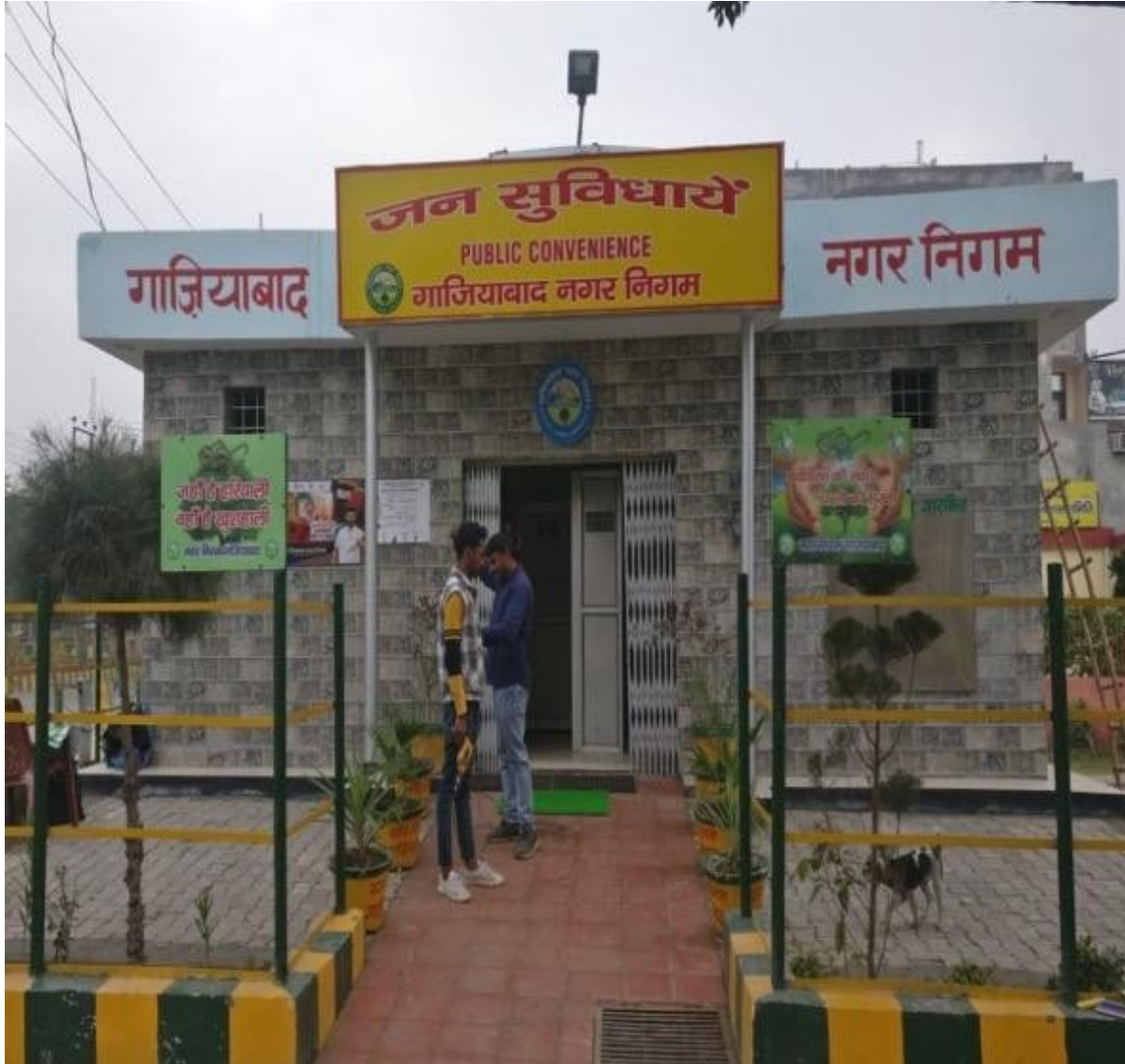
Photograph of Public toilet
