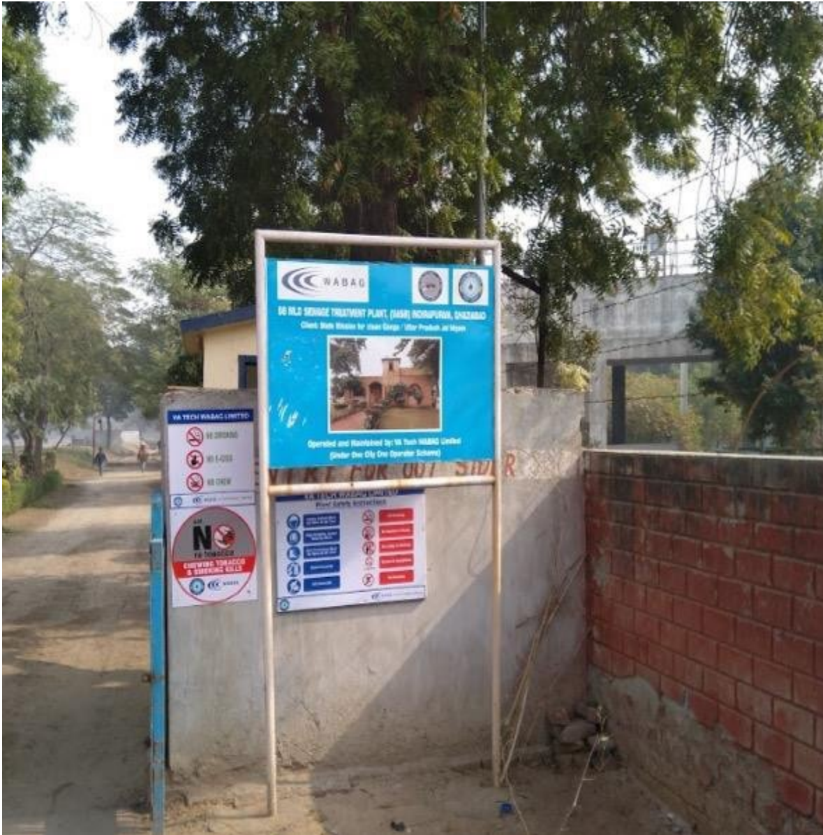
Photograph of Signage of STP plant
