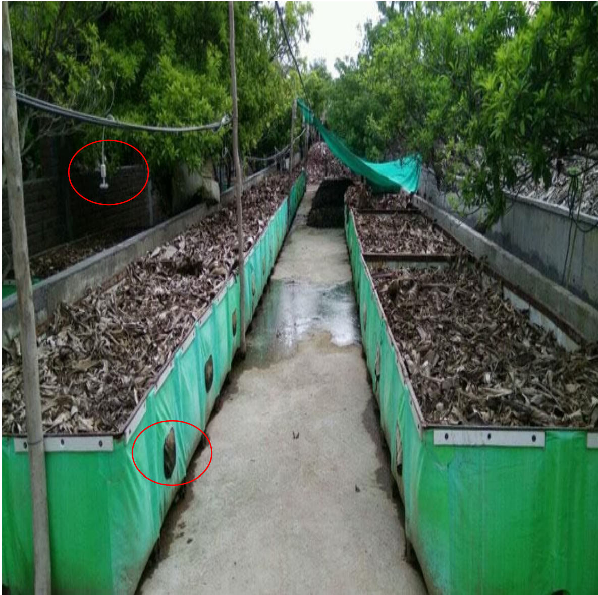
Photograph of Composting facility
